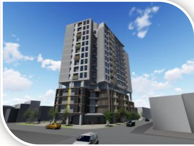
Taipei Nangang Chung-Nan Section Public Housing
